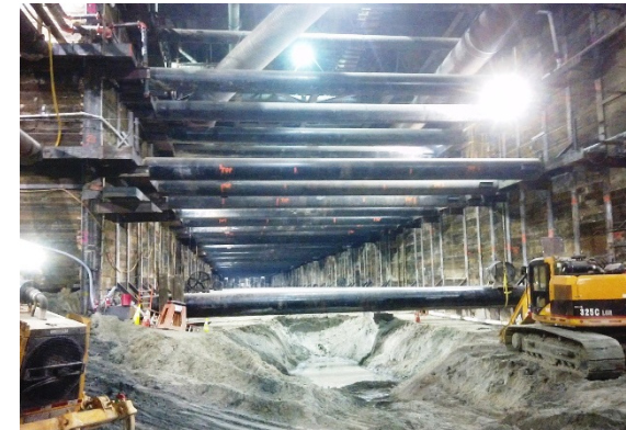
Under Deck Excavation at Wilshire/La Brea Station
