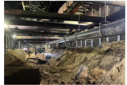
Century City Constellation Station Box Excavation
