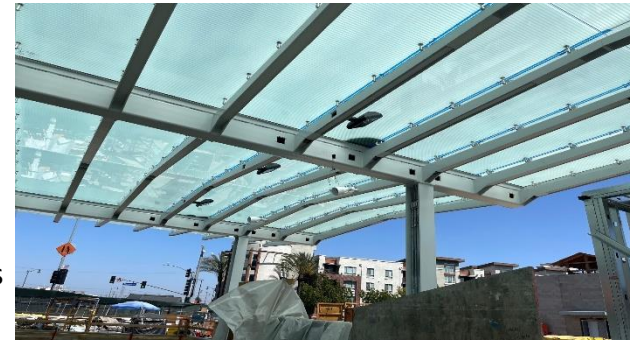
Plaza Canopy at Little Tokyo/Arts District Station
