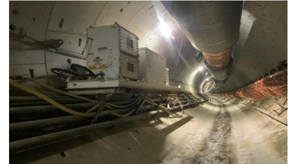
BL Tunnel Booster Fan & Transformer Installation
