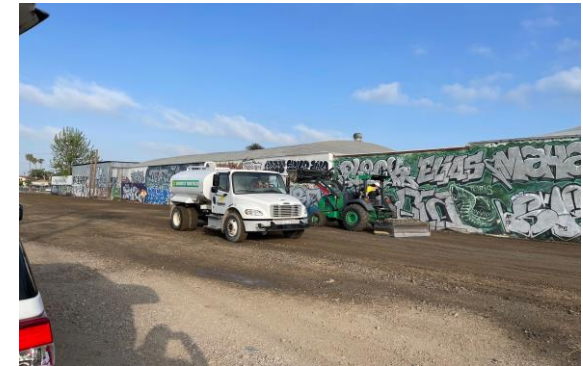
Site preparation work
