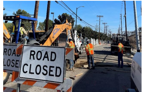
DWP Sylmar Undergrounding
