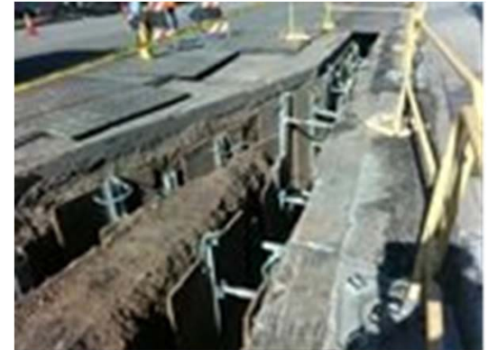
SCE Ductbank Trench Shoring
