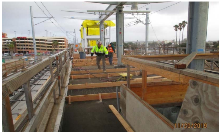
Setting forms for the platform topping slab at Aviation/Century Station
