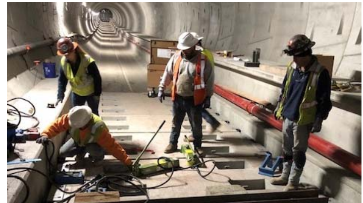
Floating Slab Track installation
