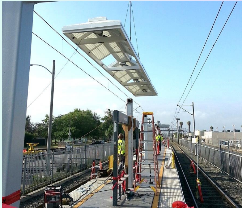
Installing new canopy at Florence Station
