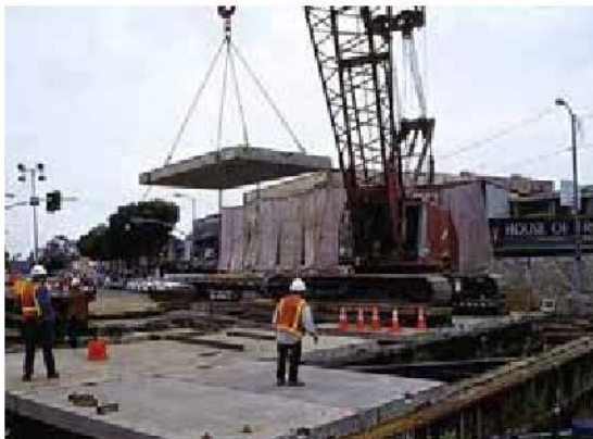
Figure 3-4: Installation of Decking (1 of 2)
