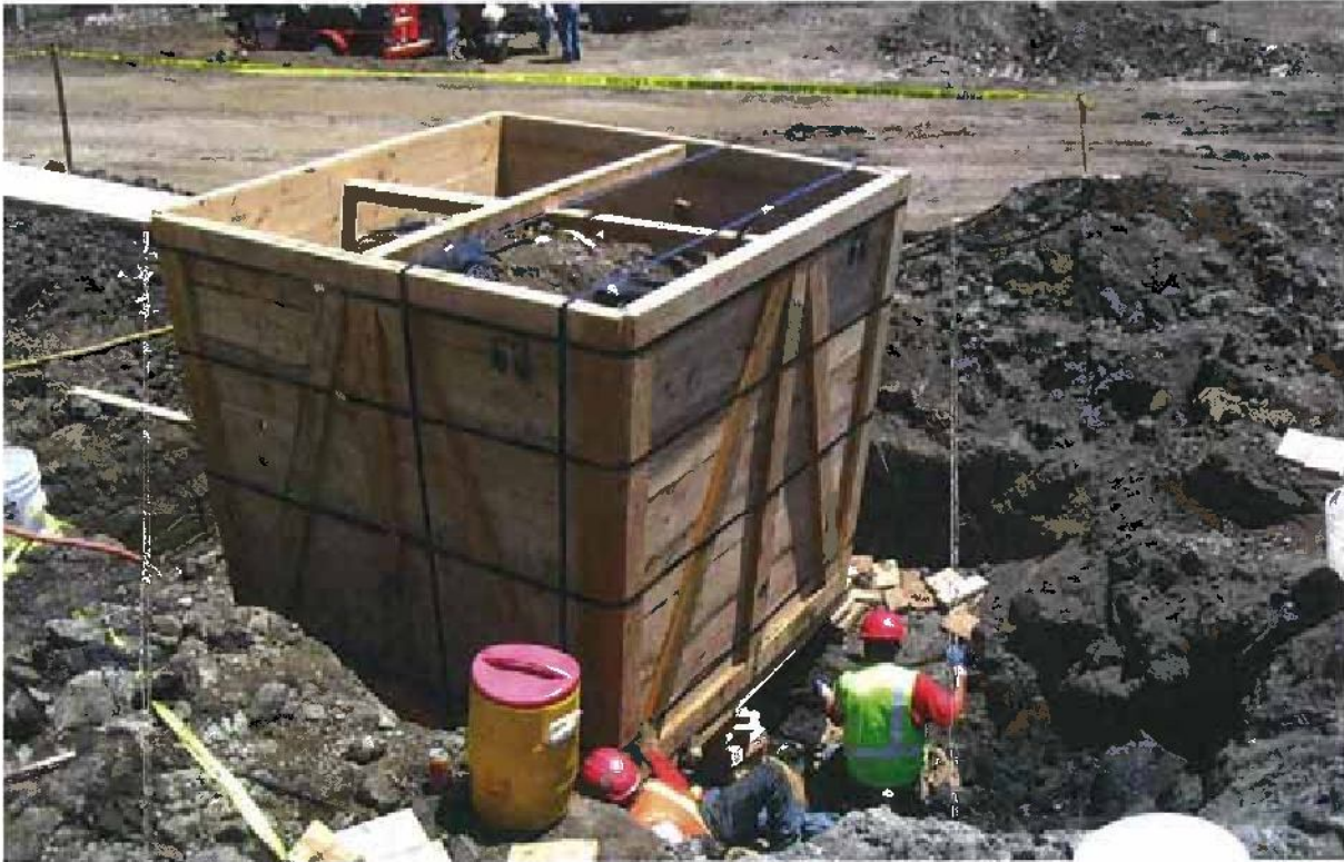
Fig 10: Tunnel under the tree box
