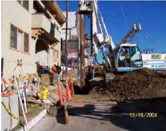
Figure 3-7: Pre-augering for Soldier Pile
