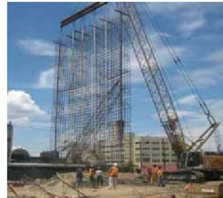
Figure 3-13: Steel Reinforcement Cage for Slurry Wall
