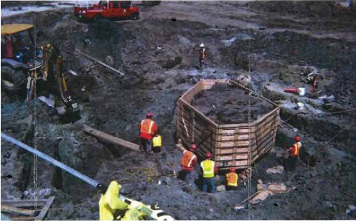
Fig 9: Secure the tree box with metal bands
