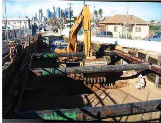
Figure 4-12: Hydraulic Excavator between Struts
