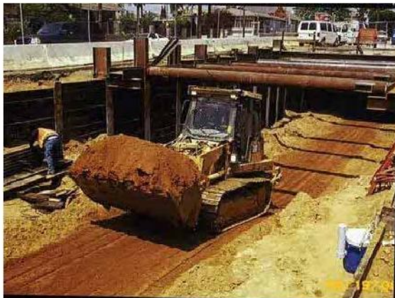
Figure 4-13: Track Loader beneath Struts
