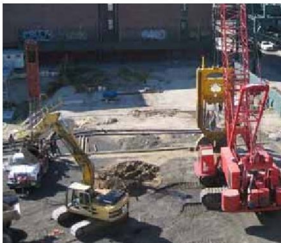
Figure 3-14: Slurry Wall Construction Equipment
