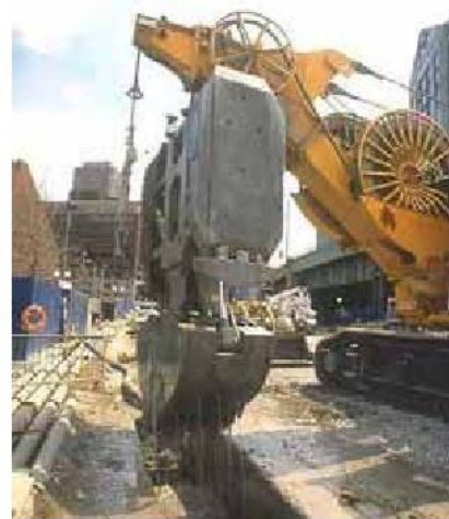
Figure 3-15: Clamshell Digger for Slurry Wall Construction
