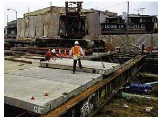
Figure 3-5: Installation of Decking (2 of 2)
