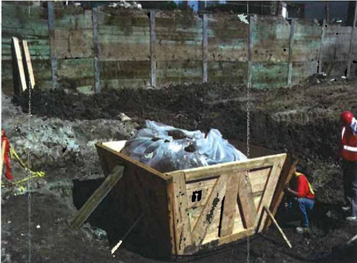
Fig 8: Building a tree box around a fossil deposit
