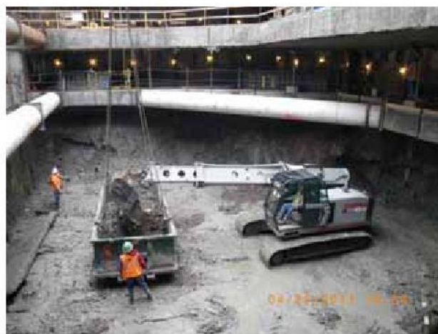
Figure 4-6: Gradall Excavator - East Side Access Project NYC
