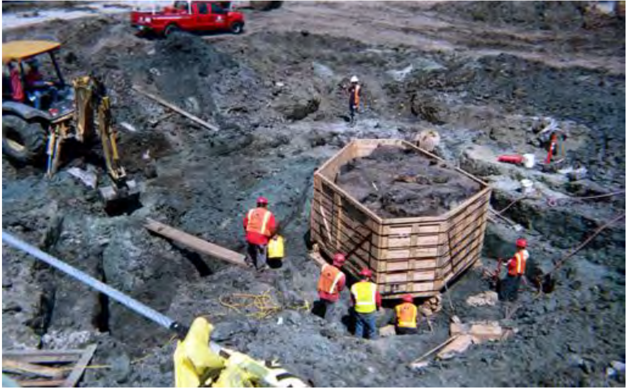
Fig 9: Secure the tree box with metal bands
