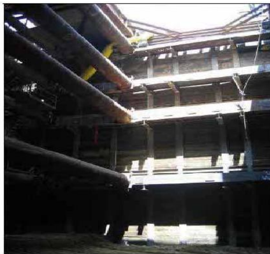
Figure 3-9: Soldier Pile and Lagging
