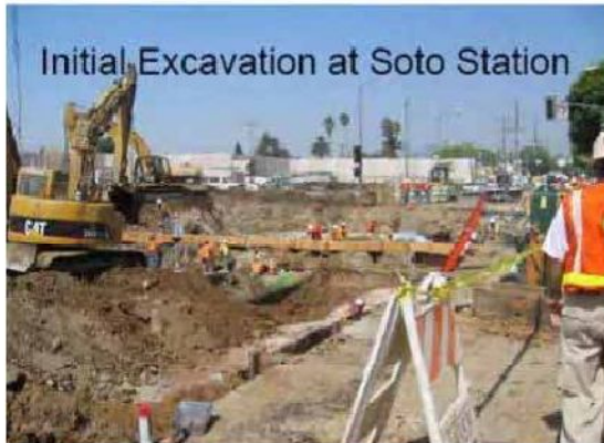
Figure 3-2: Initial Excavation at Soto Station
