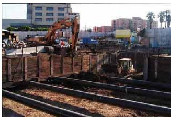
Figure 4-5: Open Cut Excavation of Side Access Shaft
