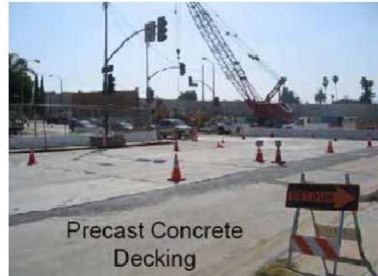
Figure 3-3: Precast Concrete Decking
