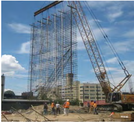
Figure 3-15: Steel Reinforcement Cage for Slurry Wall
