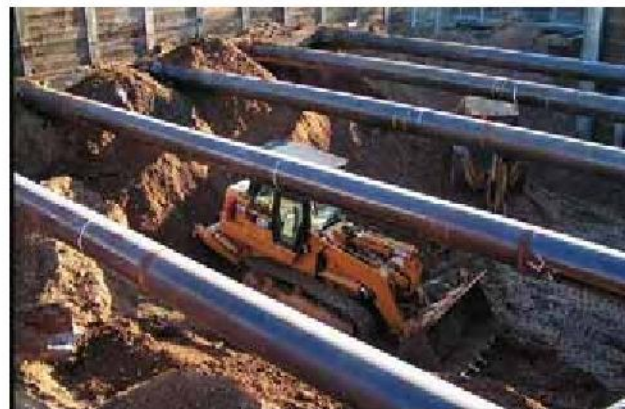
Figure 4-13: Track Loader beneath Struts
