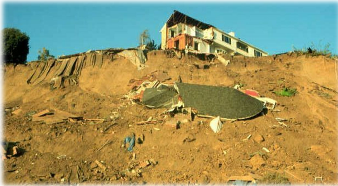
Caption: The 1994 Northridge Earthquake caused the coastal bluff under this home in Pacific Palisades to undergo a landslide, causing half the home to be torn and fall down the slope.
