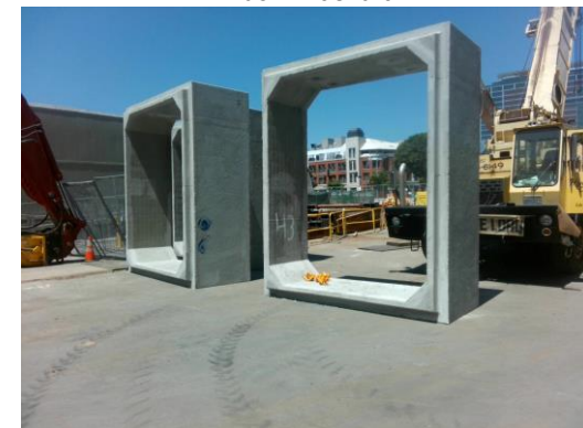
Reinforced Concrete Boxes for Storm Drain Relocation
