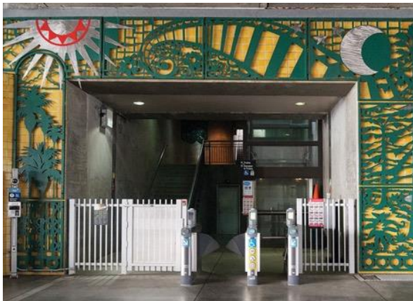
Allen Station Before
