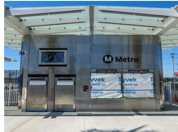
Downtown Inglewood Station – Ticketing vending machine canopy structure
