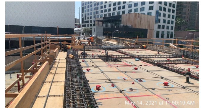
PVC and device boxes in Ped Bridge Pavilion Deck at Hope St
