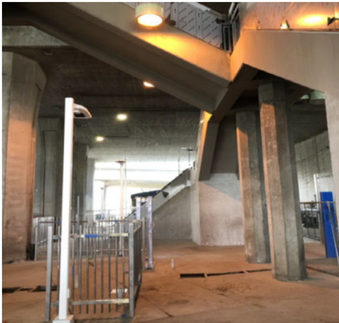
Completed concrete work @ C Line west
