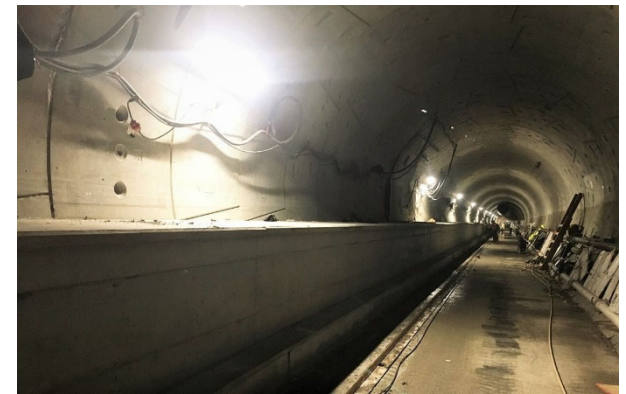
Reach 1 Tunnel Invert & Walkway Concrete Placement
