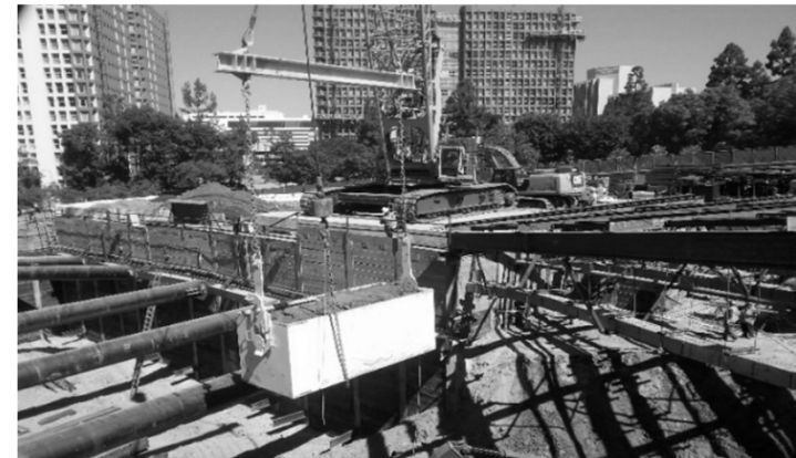
Muck Removal at 2 nd /Hope Station
