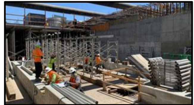
Aluminum shoring installation for roof deck at the future
