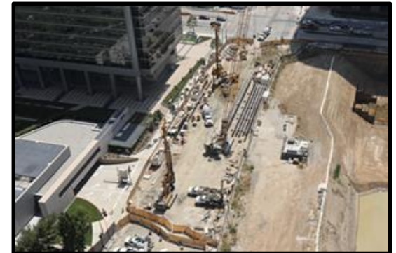
Pile installation west of the launch box in Century City
