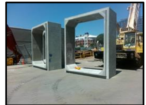
Reinforced concrete boxes for storm drain relocation.
