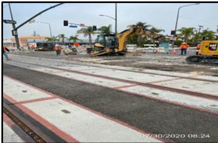
Excavating/removing section of pavement for restoration on southbound Crenshaw Blvd. and 54 th St.
