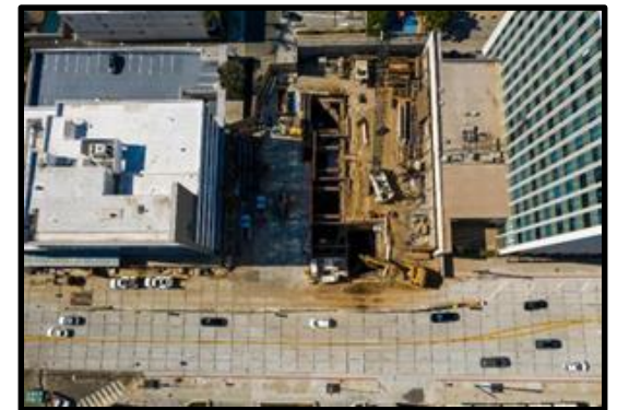
Excavation of station entrance in Beverly Hills
