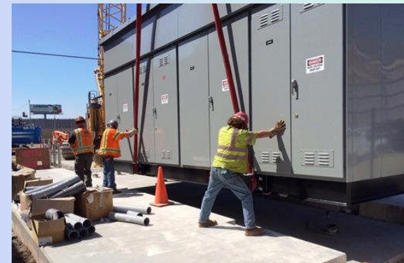
Electrical Metering Switchgear for Tunnel Operations
