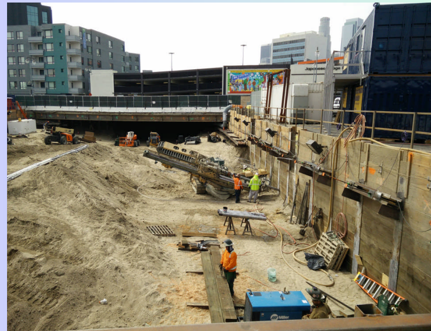
Excavation and tieback activities at 1 st /Central Station
