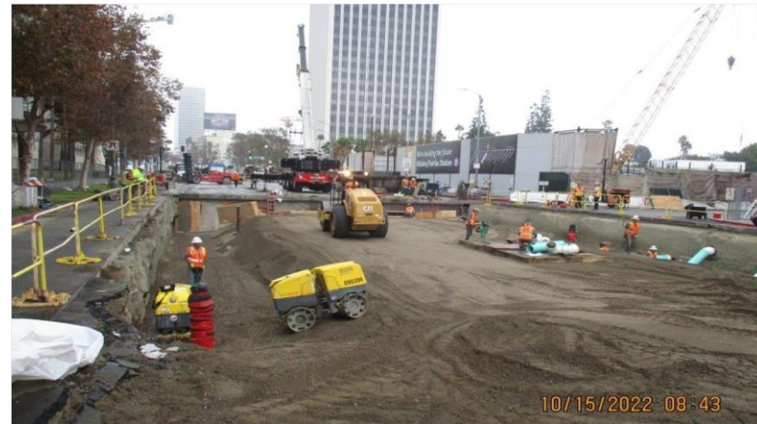
Wilshire/Fairfax Weekend Street Restoration Work
