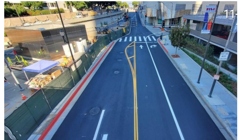
Final asphalt concrete paving along Hope St
