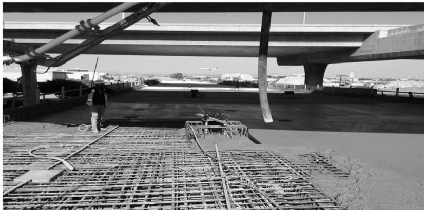
Greenline underpass deck concrete placement in progress
