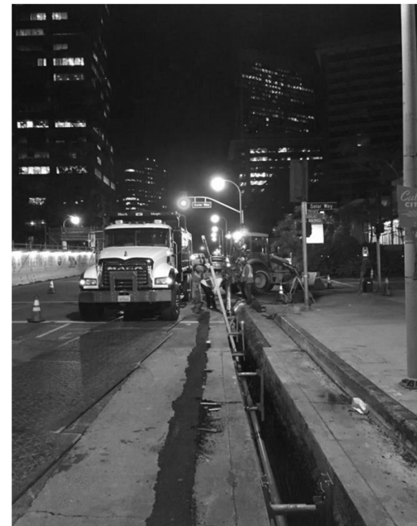
Telecom joint trench construction at Constellation Boulevard
