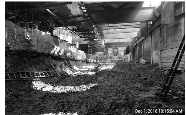
Utility hanging within 2 nd /Broadway excavation
