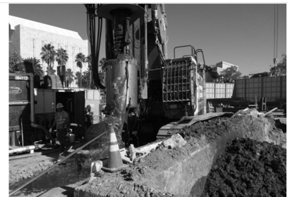
Drilling Piles at Ogden Yard
