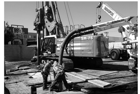
Pile installation activities at Wilshire/Fairfax Station
