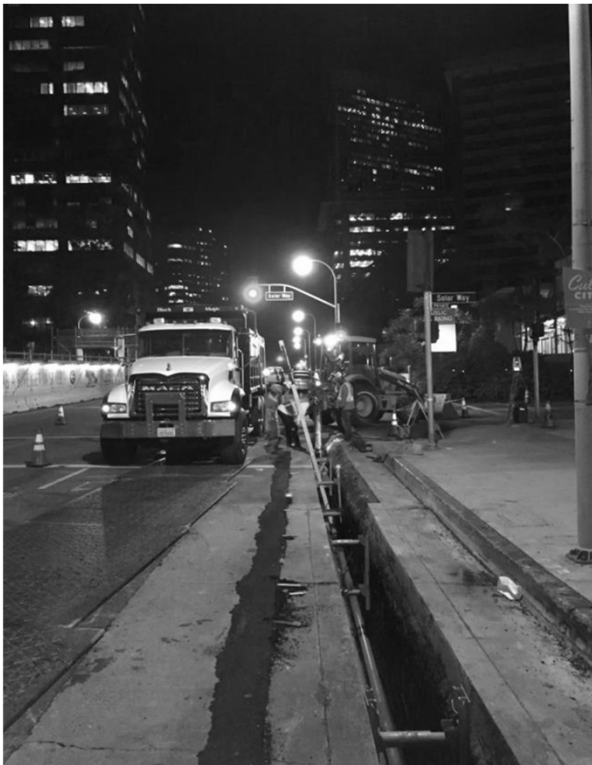
Telcom joint trench construction in Constellation Boulevard
