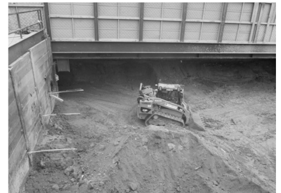
Excavation of north muck shaft Wilshire/La Brea Station
