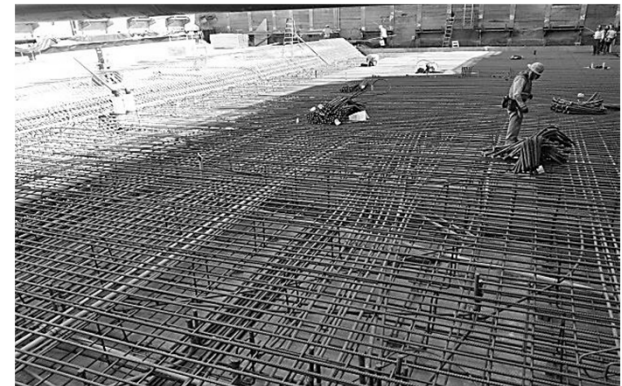
Installation of top mat of rebar and conduits for station invert at 1st/Central
