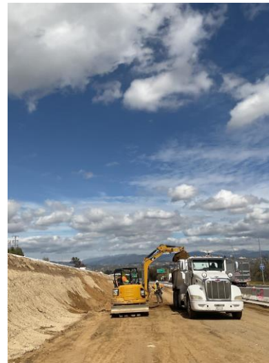
Structural Excavation for RW-2708
