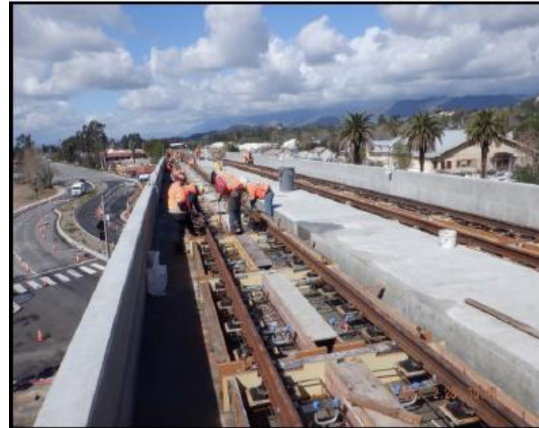
Bonita / Cataract – Structure Track Direct fixation
