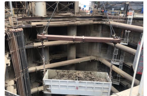
Tunnel Muck Removal in Century City
