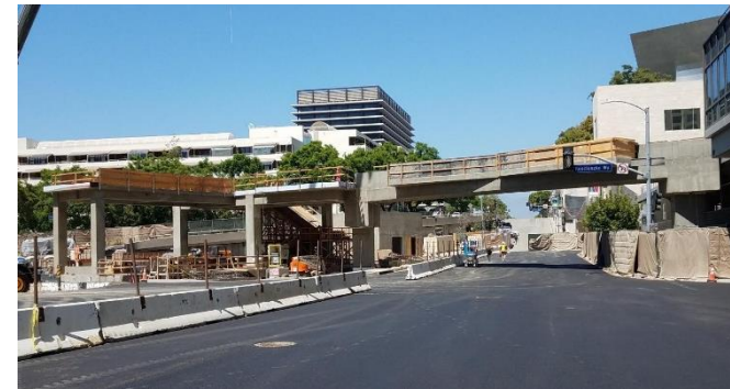
Asphalt pavement complete along Hope Street
