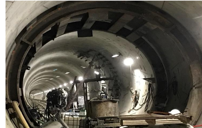
Reach 2 Cross-Passage Excavation Preparation
