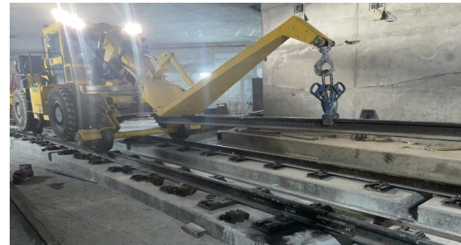
1st Street Leg Plug Rail Installation
