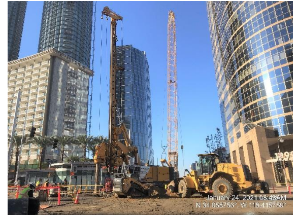
Pile Installation on Constellation & Avenue of the Stars
