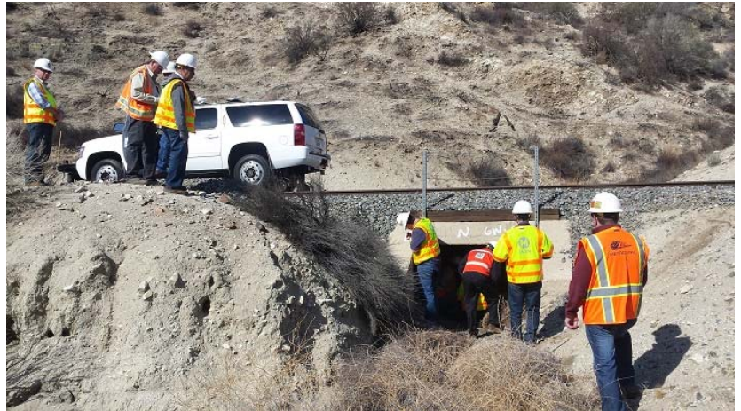
Picture 6: SCRRRA and MTA Staff inspecting a "Rail-Top" Bridge on the Valley Subdivision
