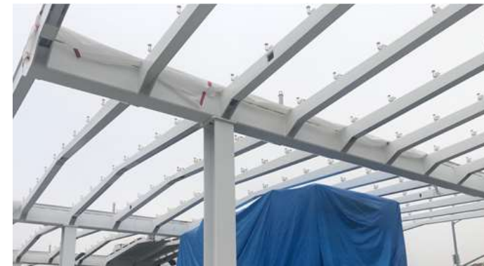
Little Tokyo/Arts District Station Canopy Installation
