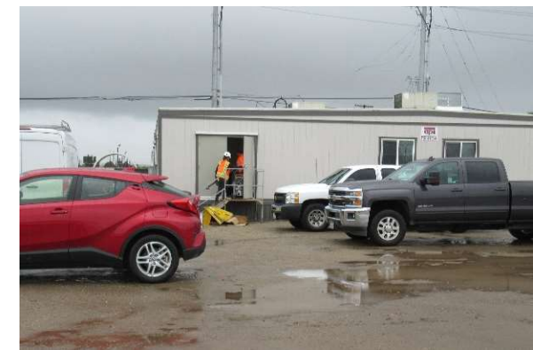
Mobilization for Main Station Construction
