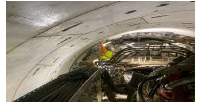
Ring Installation in the BL Tunnel
