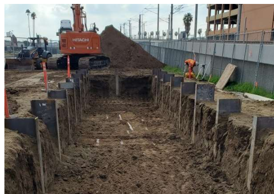
Shoring in progress
