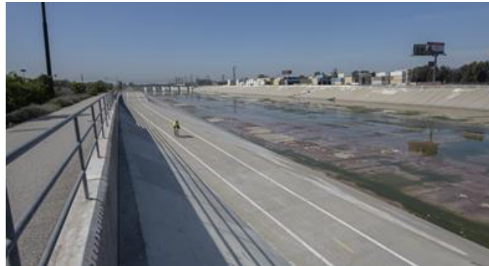
Figure ES-1: LA River Bike Path (South Bay Section)
