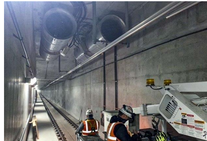
UG3 contractor performing mechanical testing on tunnel booster fans
