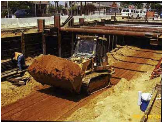
Figure 4-13: Track Loader beneath Struts
