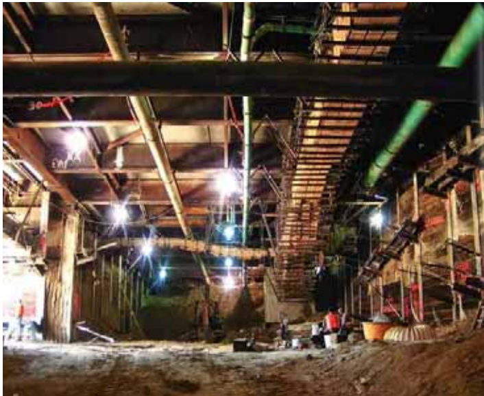
Figure 3-17: Utilities Hung from Deck Beams
