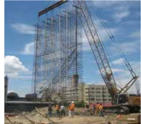
Figure 3-13: Steel Reinforcement Cage for Slurry Wall
