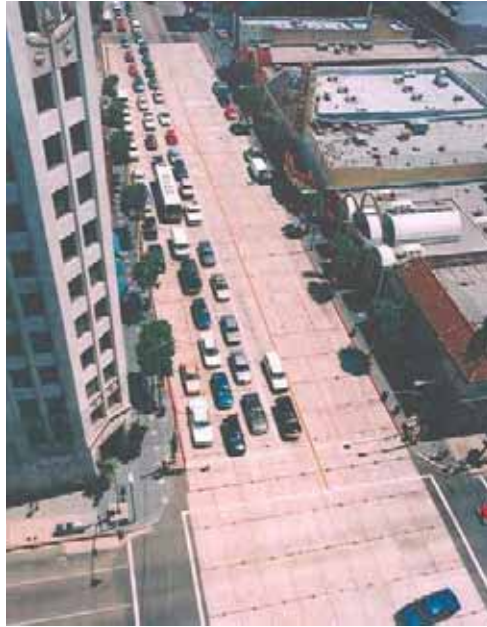
Figure 3-6: Roadway Operations Restored on Temporary Decking System
