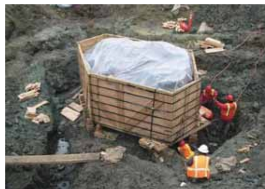
Figure 4-2: Fossil Box Construction at Project 23
