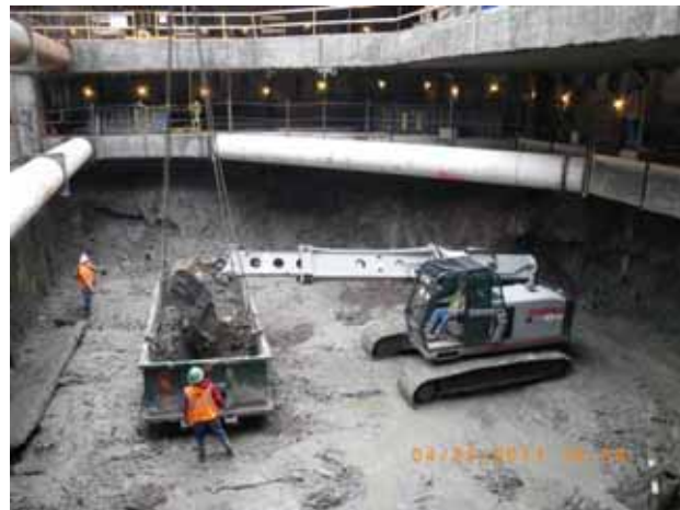
Figure 4-6: Gradall Excavator - East Side Access Project NYC
