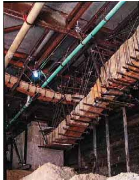
Figure 3-18: Utilities Hung from Deck Beams (Close Up)
