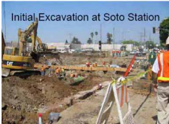
Figure 3-2: Initial Excavation at Soto Station
