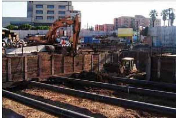
Figure 4-5: Open Cut Excavation of Side Access Shaft
