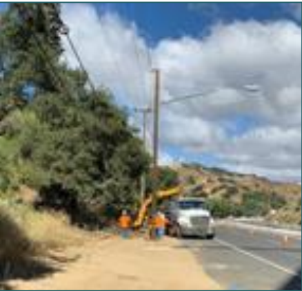
Old Road-SCE Power & AT&T Relocation
