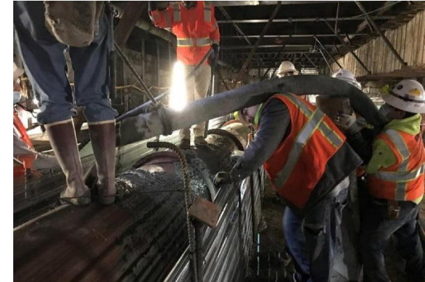
Wilshire/La Brea Concrete Placement Above Station Roof
