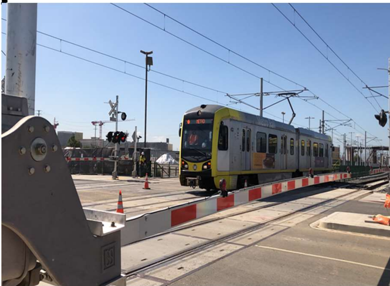
Testing crossing gates with train at Arbor Vitae Street
