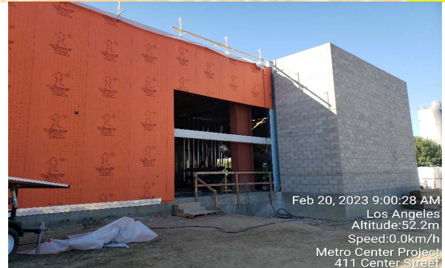
Exterior Finish – Weather Barrier & Sheet Metal
