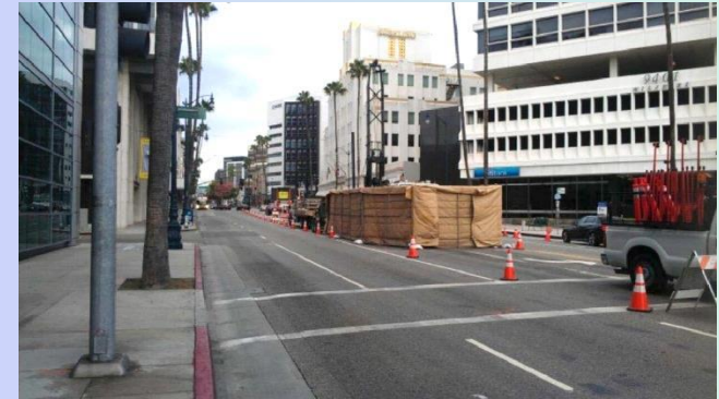
Geotechnical Drilling on Wilshire at Reeves
