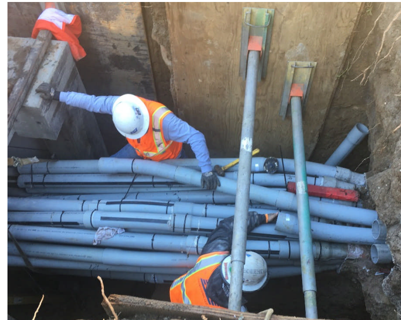
AT&T Conduit Installation in Century City
