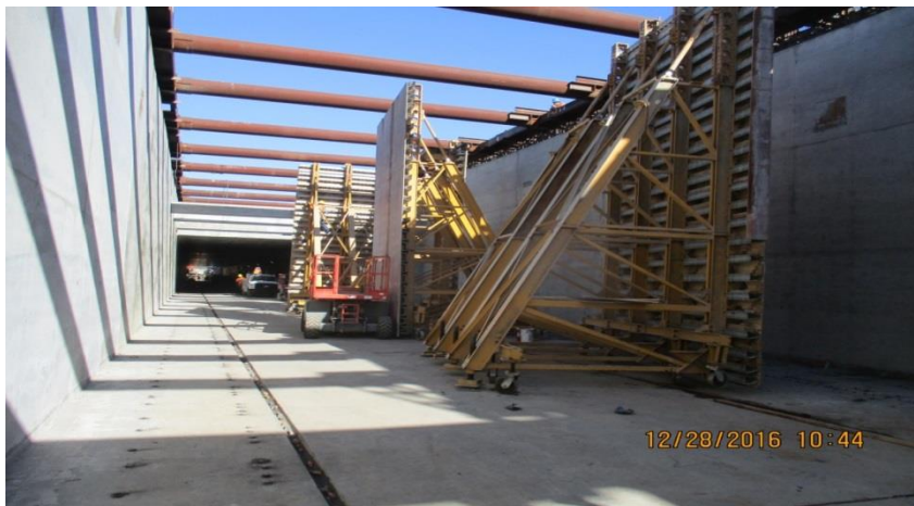
Underground guideway No. 1 open cut at struted u-wall
