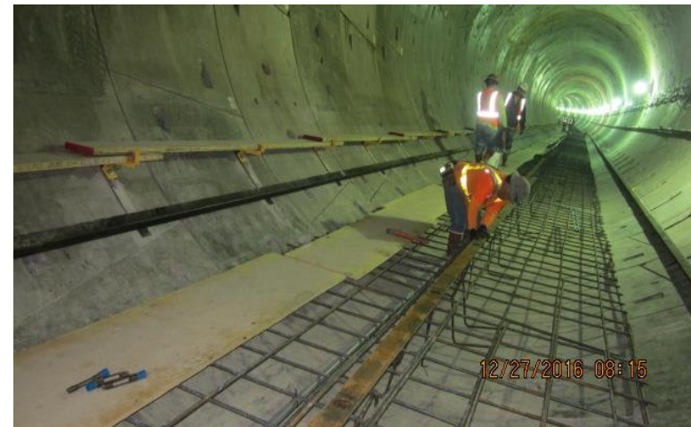
Initiating southbound tunnel concrete invert work
