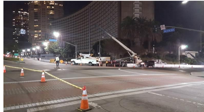
Telecom joint trench construction at Constellation Boulevard
