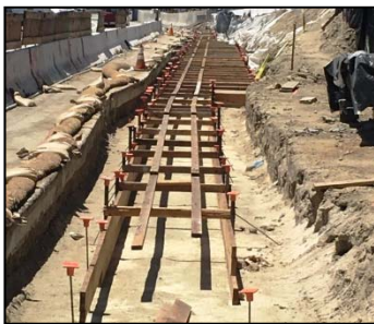
Retaining wall located near features requires no further excavation
