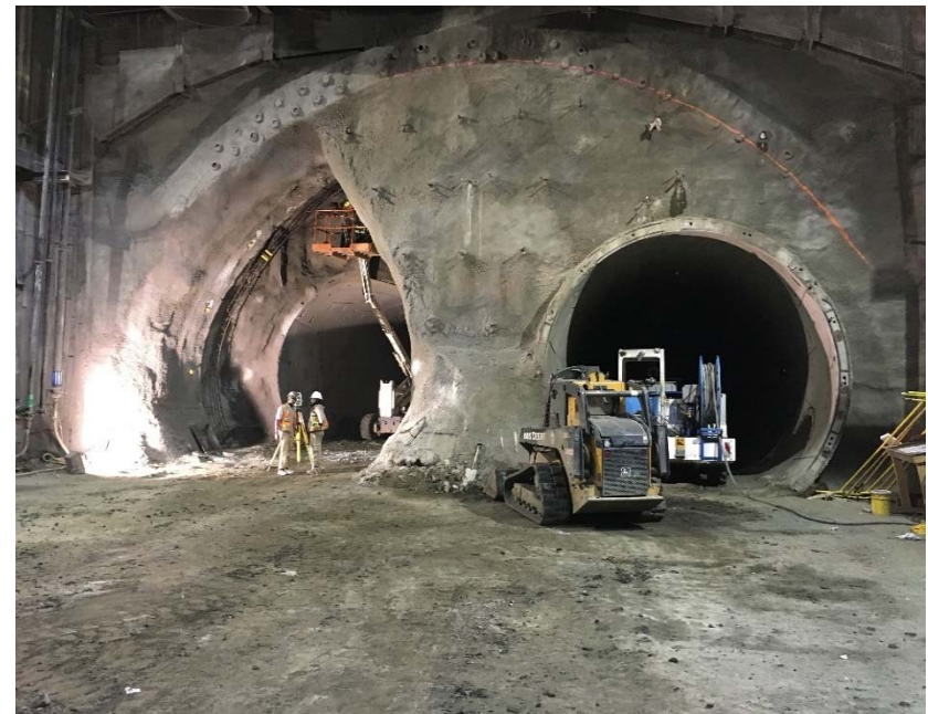
Sequential Excavation Method (SEM) in Historic Broadway Station
