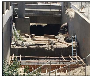
Elevator foundation on Metro R/W requires only forming and concrete pour
