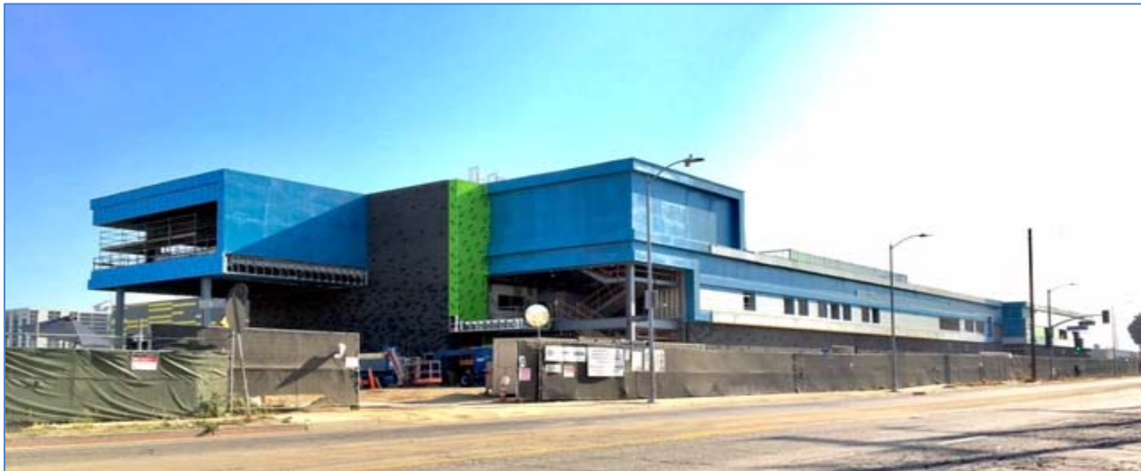
Continuing construction of main shop building at Southwestern Yard Maintenance Facility
