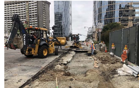
AT&T Utility work in Century City
