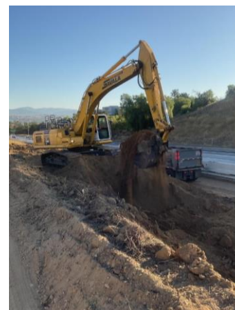
Median Excavation work for retaining walls in progress
