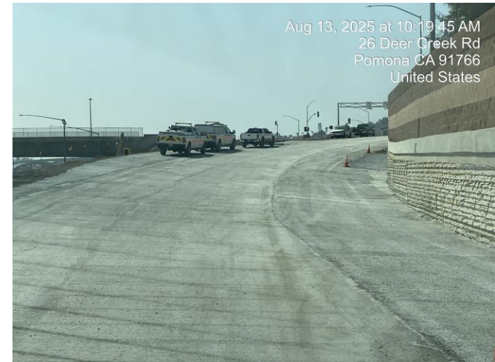
Realigned SB Rio Rancho off-ramp, LCB paving.
