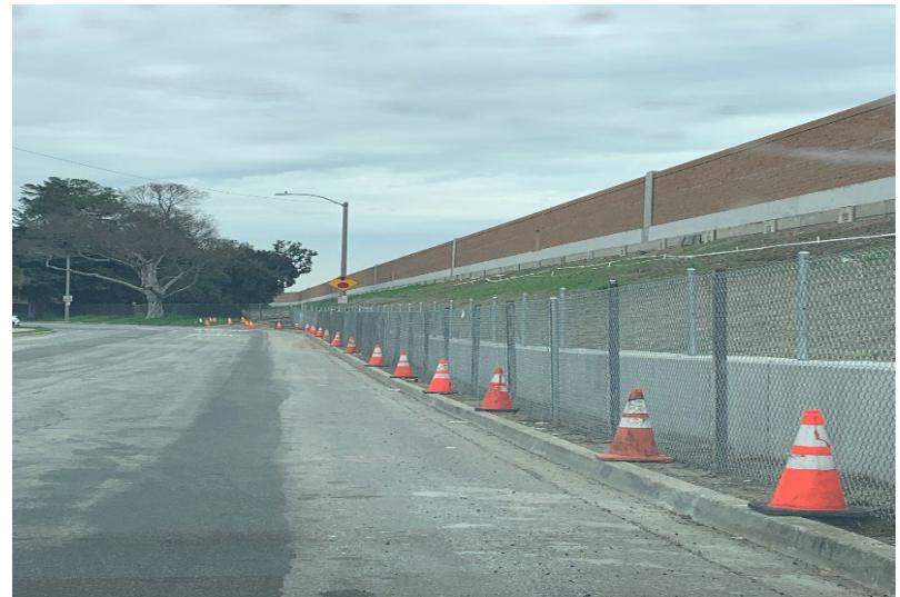
NB 405 South of Van Ness Blvd (SW #760) with completed retaining concrete barrier at 186 th Street
