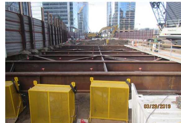
Installed Deck Beams
