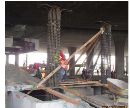
Pile work at Blue Line Platform
