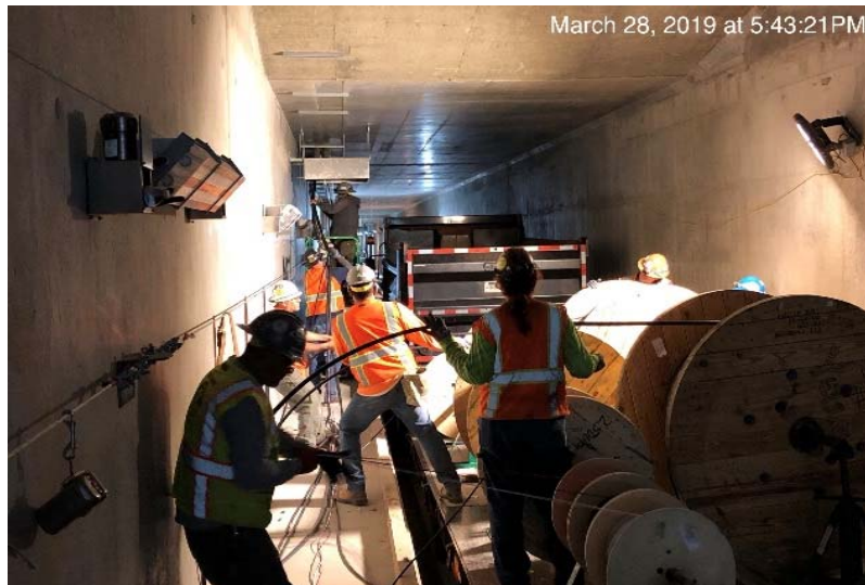
Installing electrical conduit in underground tunnel
