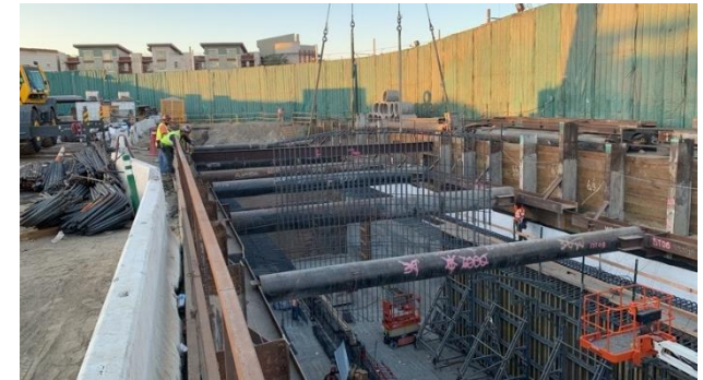
Exterior wall segment installation at Alameda Leg
