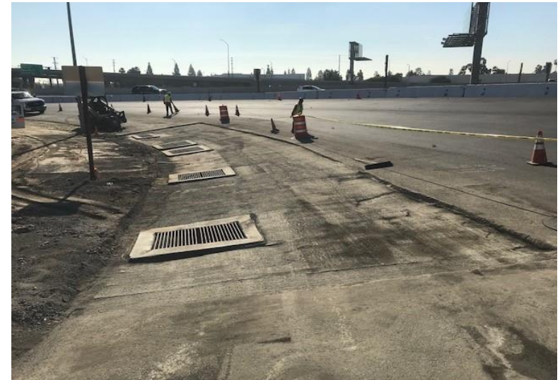
Northbound Valley View offramp
