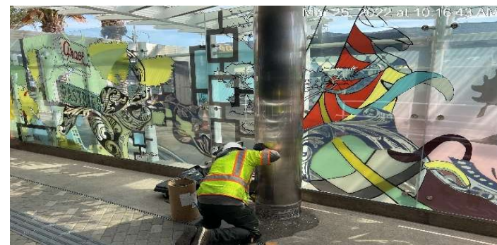
Hyde Park Station – Applying anti-graffiti shield
