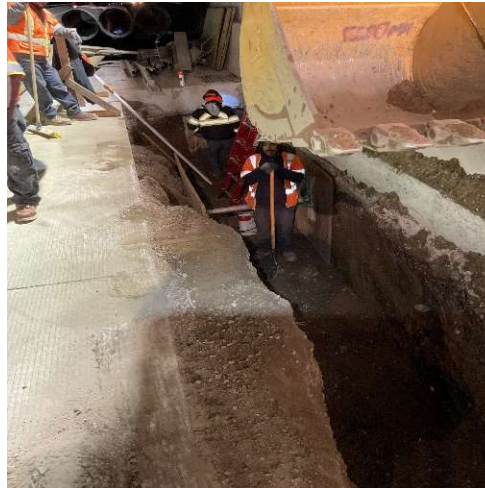
Drainage excavation on SB I-5 median DS# 159
