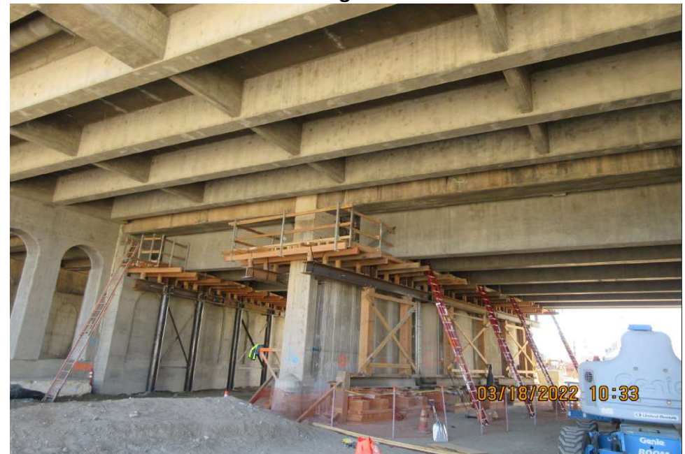
1 st Bridge – Bent 16
