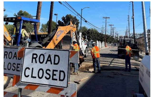
DWP Sylmar Undergrounding
