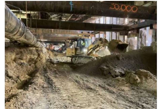
Century City Constellation Station Box Excavation
