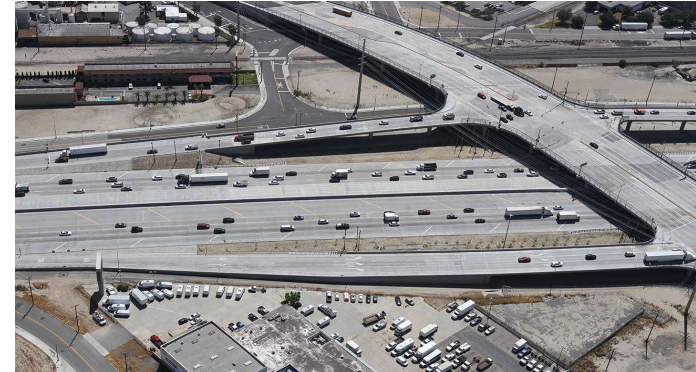
I-5 South/Carmenita Interchange
