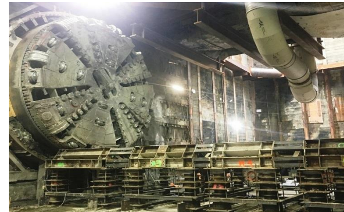
Preparations for Retrieval of TBM #1 at Wilshire/Western
