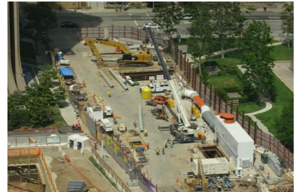
TBM Launch Box Overview in Century City
