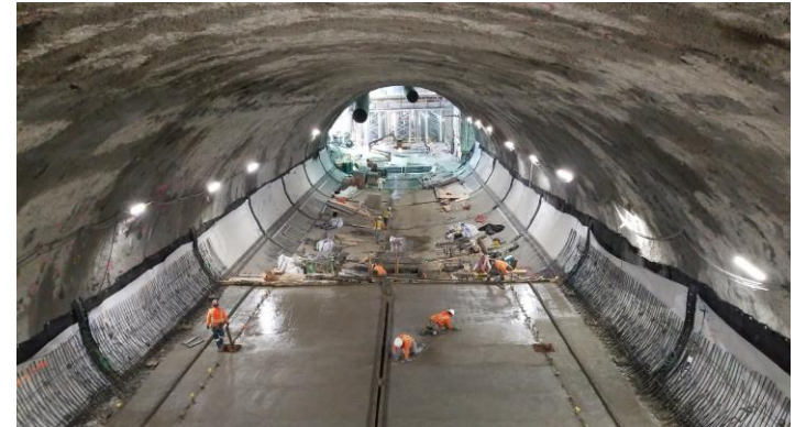
Invert placement in SEM Cavern
