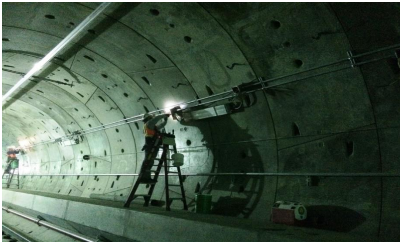
Installation of emergency lighting at southbound tunnel
