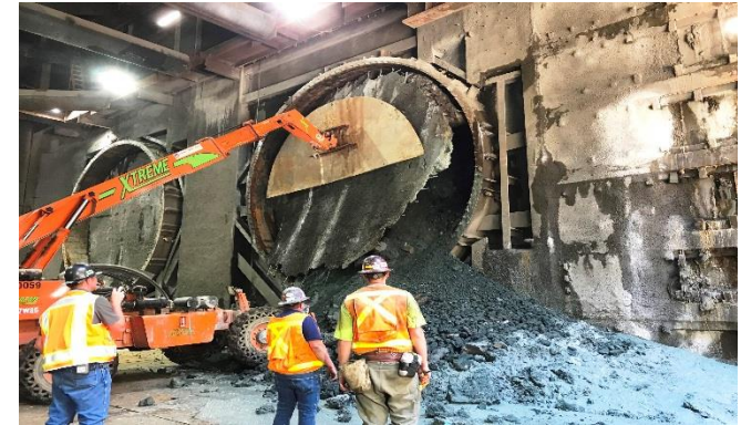
TBM #1 Break Through at Wilshire/Western
