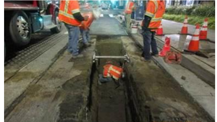
Installing Riser for Water Pressure Test
