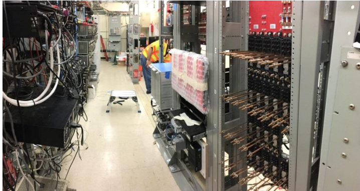
Train Control work in existing bungalow
