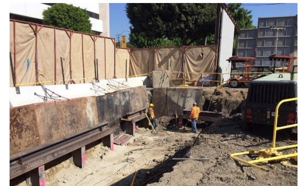
Securing Cap Beams at Wilshire/La Cienega Yard
