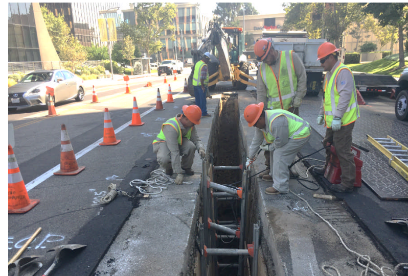
LADWP power relocation work in Century City
