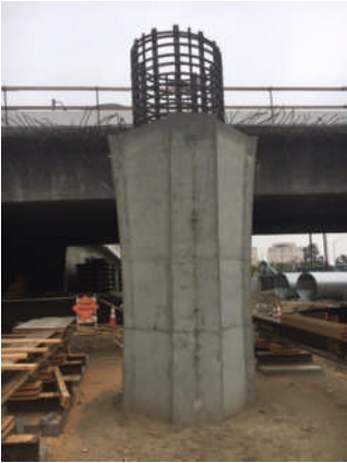
Completed bridge column
