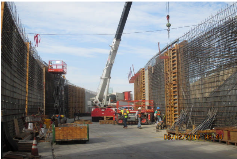
Installation of formwork for UG#3 walls south of Hyde Park Blvd.
