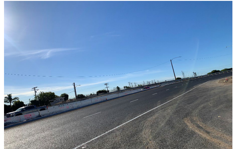
SB Crenshaw Blvd to SB 405 on ramp realignment completed
