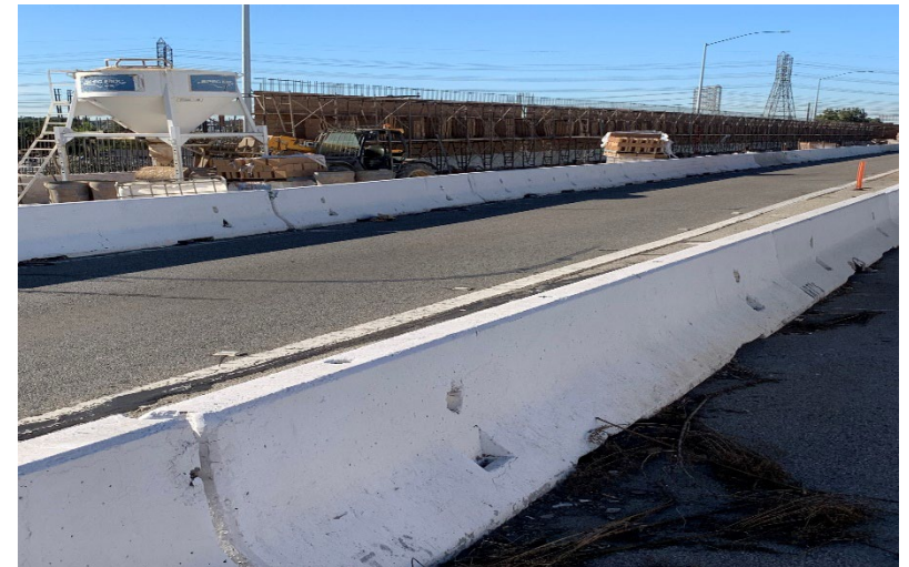
SB 405 Crenshaw Blvd off ramp (SW #815)
