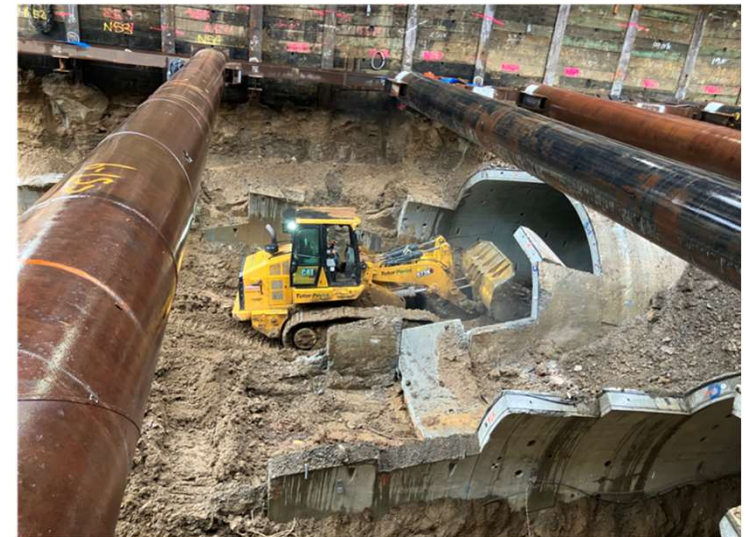
Westwood/VA Hospital Station: BR Tunnel Liner Removal in Excavated Station Box
