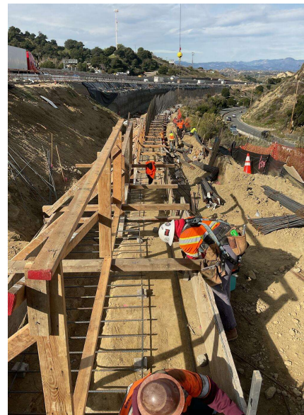
Rebar Installation at Retaining Wall 2460
