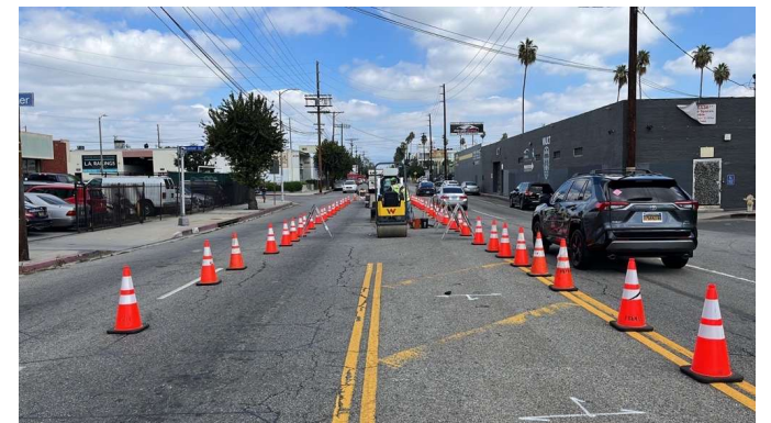
Pothole Restoration on Kester Ave
