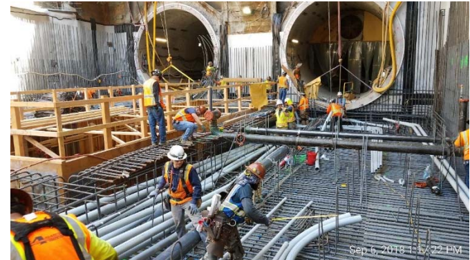
Rebar and UMP installation at Grand Av Arts/Bunker Hill Station
