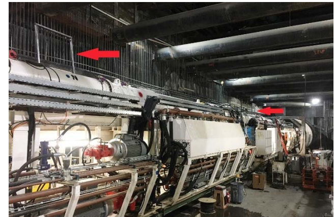
TBM Assembly at Wilshire/La Brea Station
