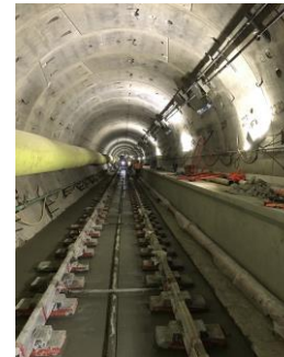
BL R4 Completed Second Stage Invert Track Concrete Pour
