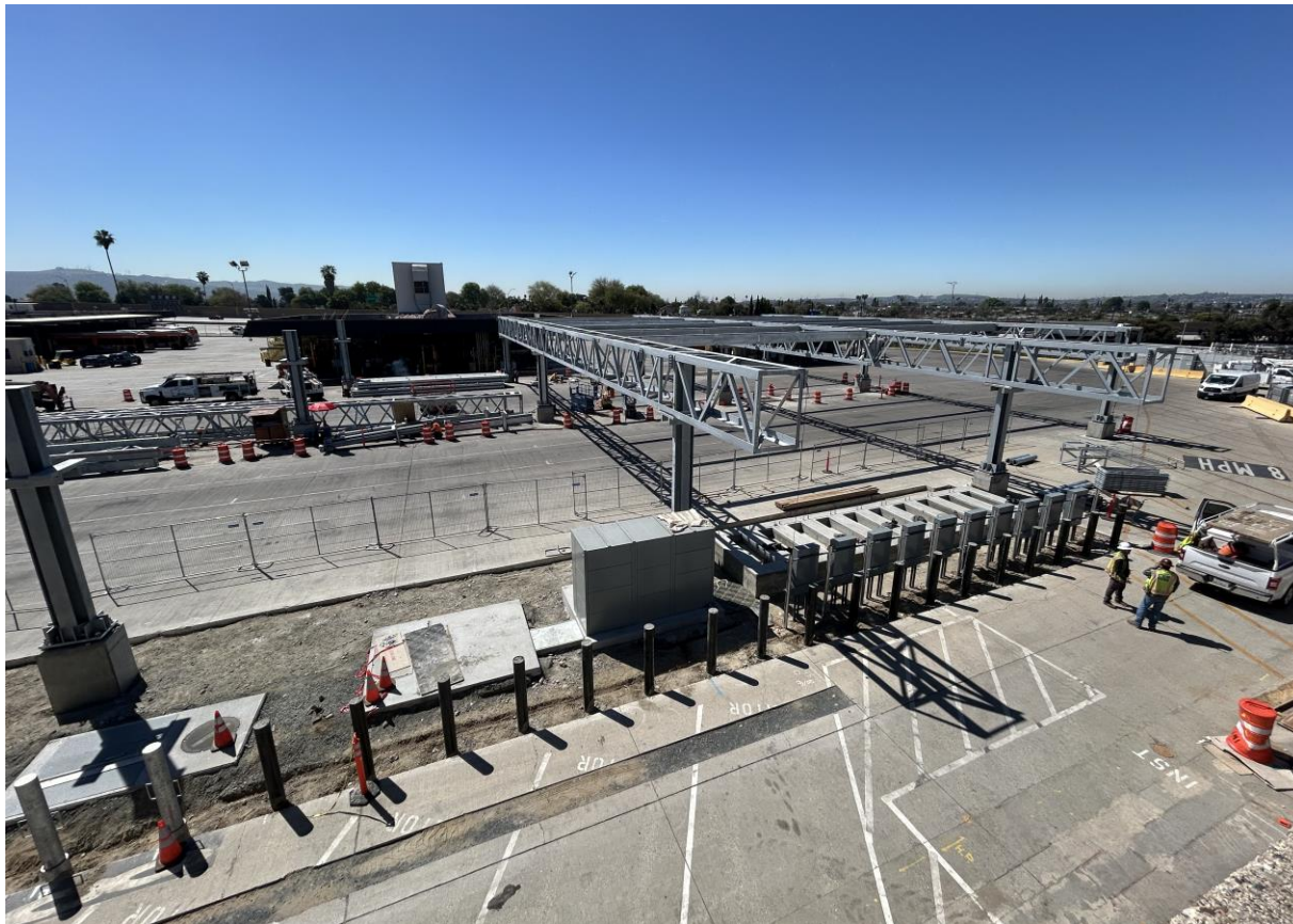
Photo: Progress at Division 9
