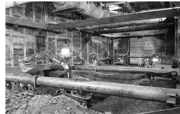
Excavation and lagging for TBM Retrieval Shaft
