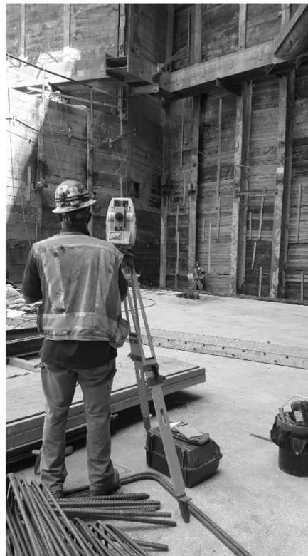
2 nd /Hope Survey for Tunnel Eye
