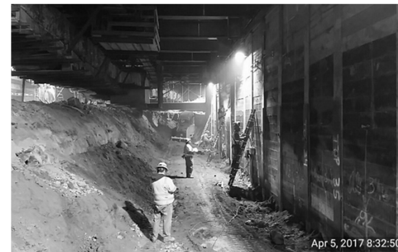
Excavation and utility hanging under 2 nd Street
