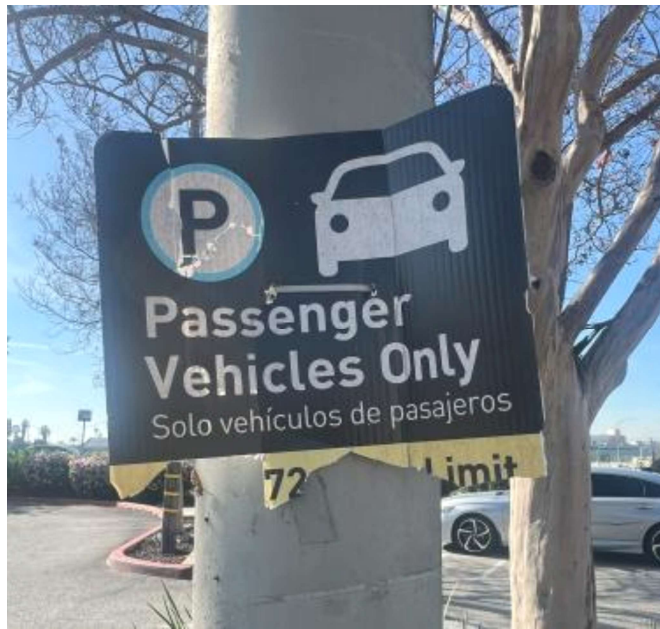
Picture 7 2/25/2026 – Hawthorne/Lennox (C Line) Torn/Damaged Sign
