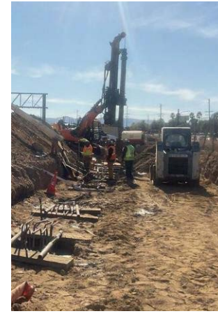
Wall 986 Installation of 24IN CIDH Piling
