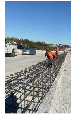
Median Barrier Rebar Installation
