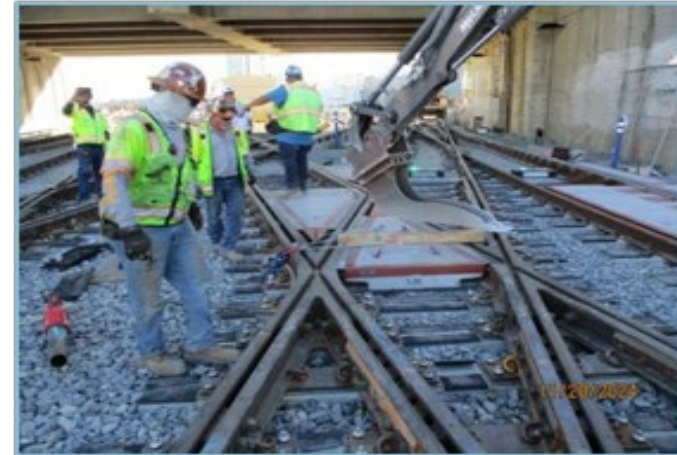
Crossing Panel Installation
