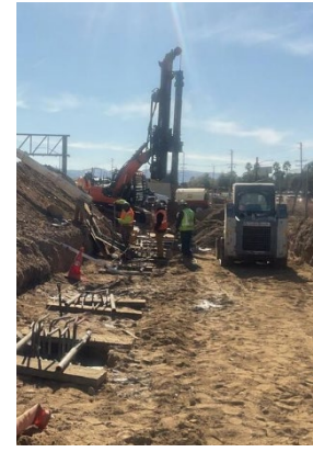
Wall 986 Installation of 24IN CIDH Piling
