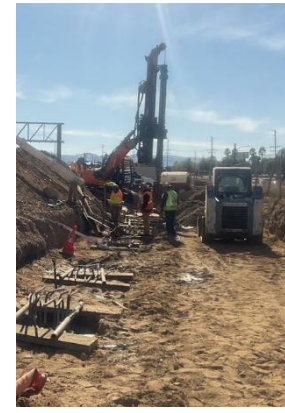
Wall 986 Installation of 24IN CIDH Piling
