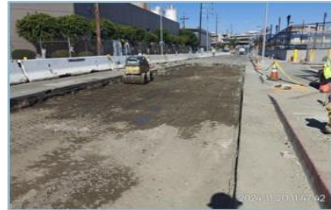
Center Street Reconstruction
