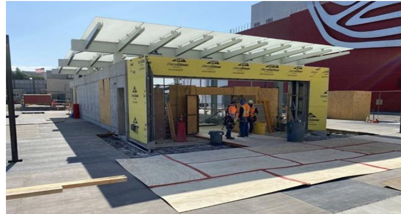
Wilshire/Fairfax Station Entrance Plaza
