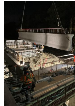
Set Girders at Rye Canyon Bridge
